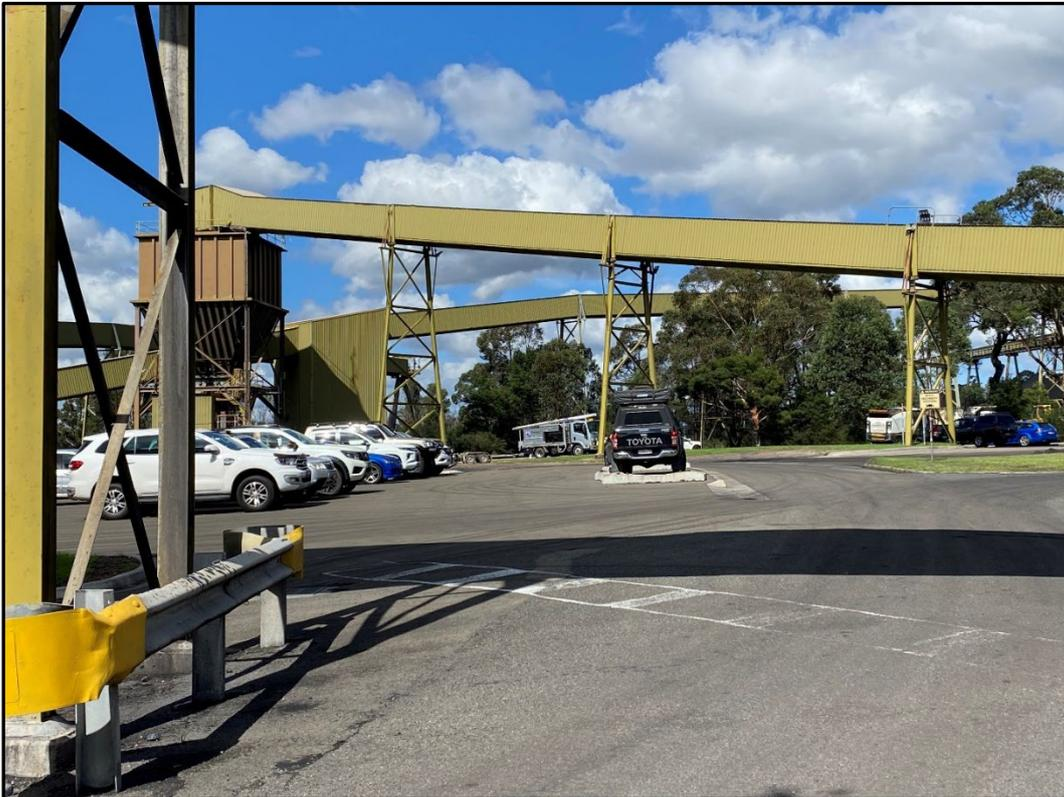
**Plate 6. Enclosed Conveyor Belts**
