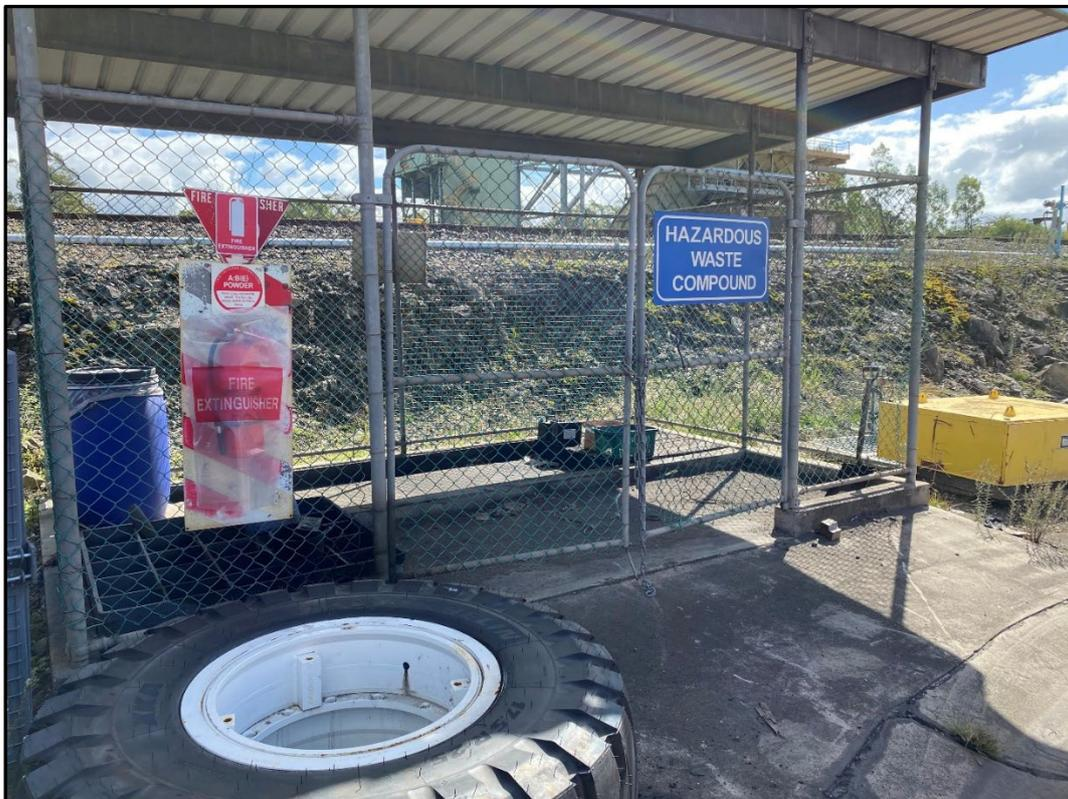
**Plate 4. Hazardous Waste Compound (Sealed, bunded roofed)**
