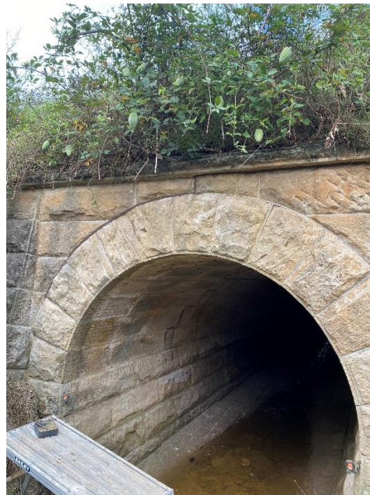
12. Downstream end completed
