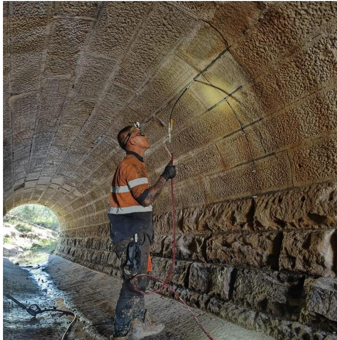
9. Epoxy crack injection
