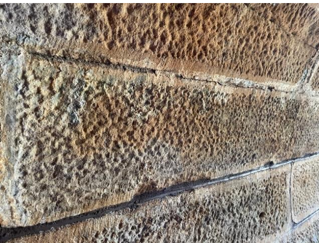
Figure 2 – Mortar repairs/replacement
