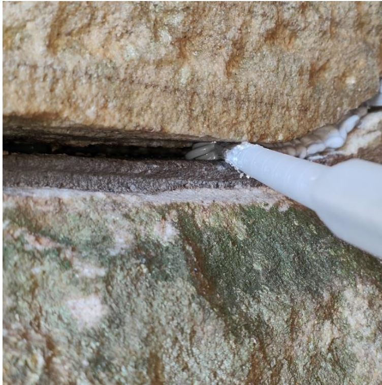
7. Sealing crack prior to injection
