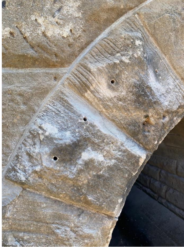
1. Cored holes in stone
