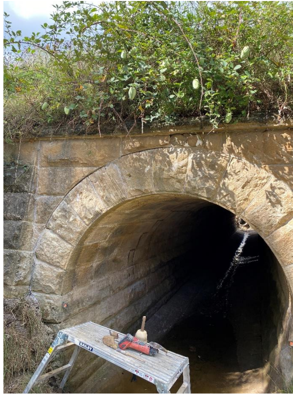
11. Downstream end during the work
