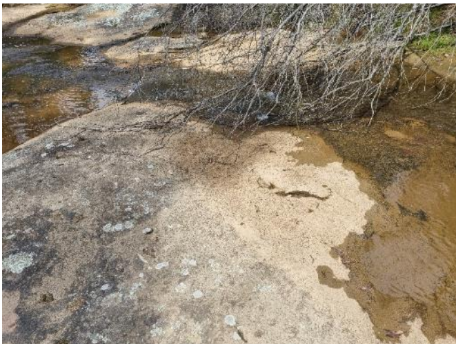
Weathering, cracking on North bank of Rockbar 2 19/10/2022
