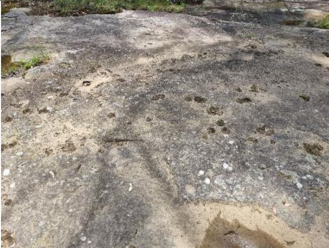
Joint on north rockbank at rockbar 2 Depression 3 Looking north 19/10/2022
