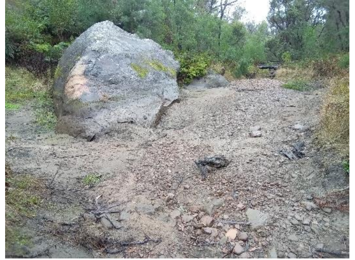
Additional Iron Staining 28/06/2023
