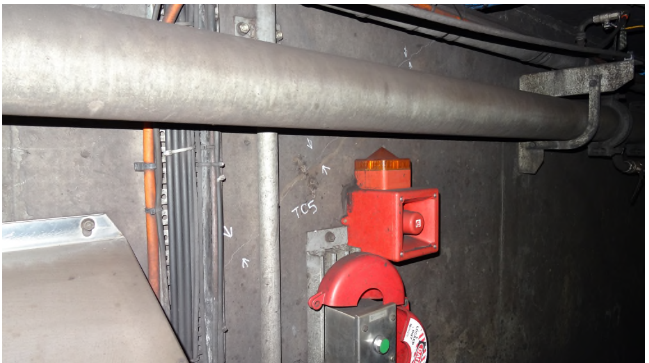
Photo 5: General location of crack C5 (Toms crack).
