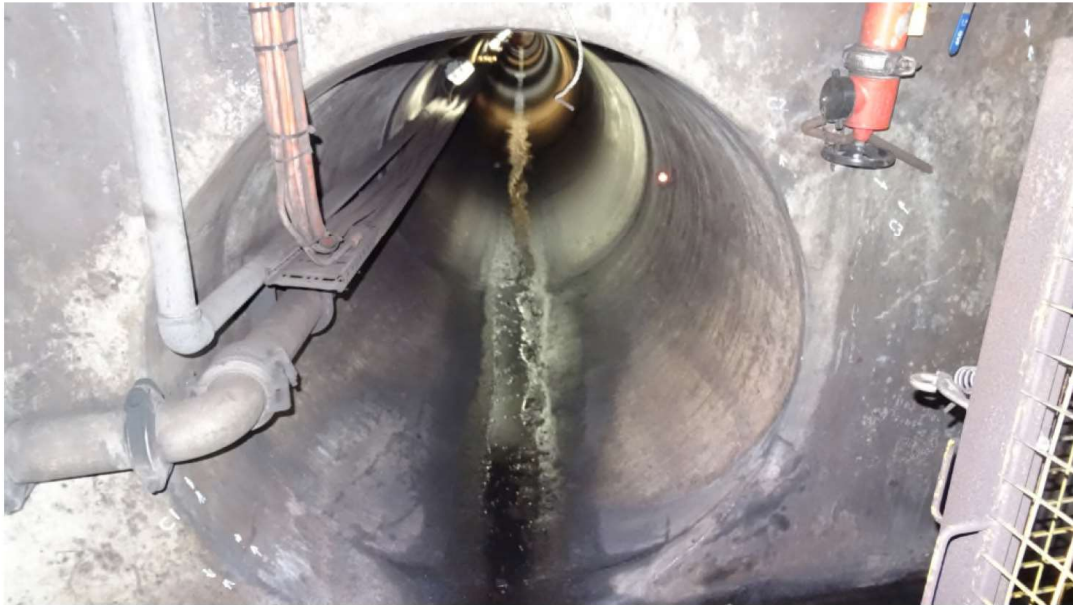
Plate 4.3 Context for the location of cracks C1, C2 and C3 (David Talbert, 6 June 2023).
