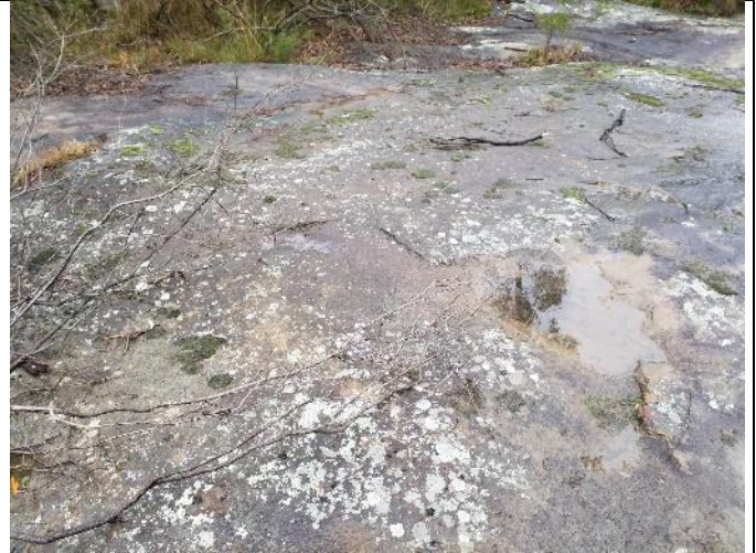
Joint on north rockbank at rockbar 2 Depression 3 Looking north 28/06/2023
