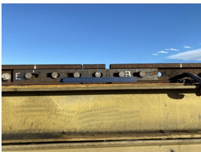
Figure 1 and 2: 5C slide joint east showing variation 13/06 to 27/06.
