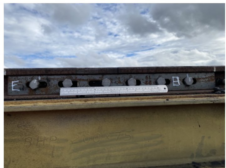
Figure 1: 5C slide joint east showing closure of gap (29/05 vs 06/06)
