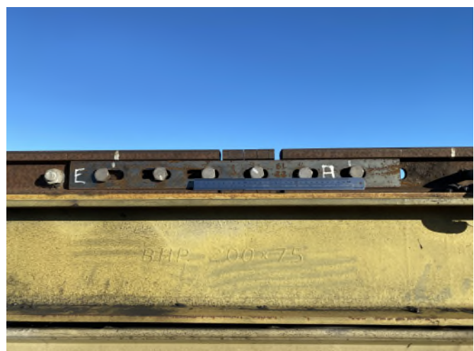
Figure 1 and 2: 5C slide joint east showing variation 13/06 to 27/06.
