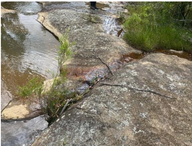
South Rockbank flowing into Depression 5 19/10/2022
