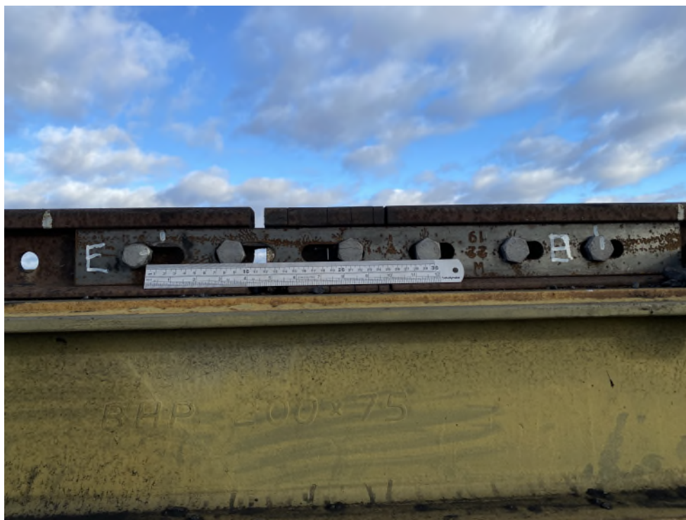
Figure 1: 5C slide joint East with spacer installed (29/05)
