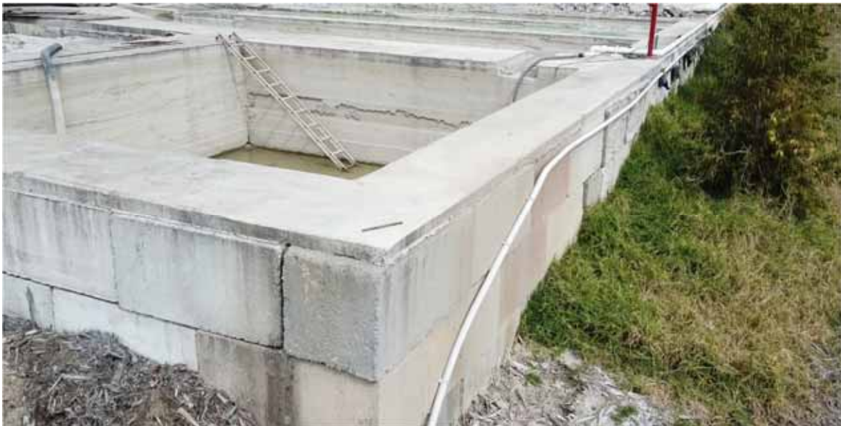
Fig. 1.6 Sedimentation ponds
