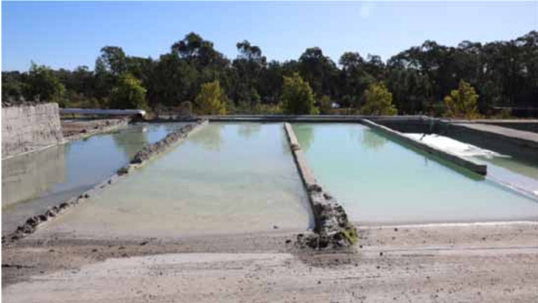
Fig. 1.6 Sedimentation ponds
