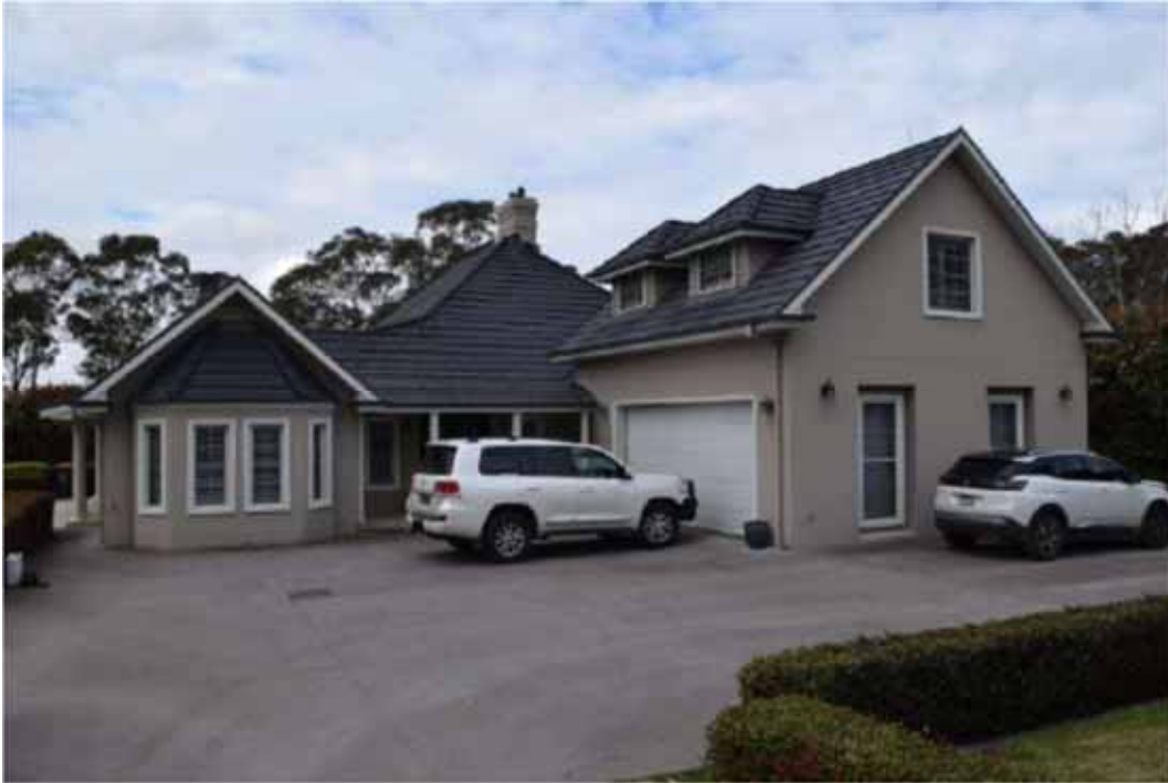
Photograph courtesy JMA Solutions
