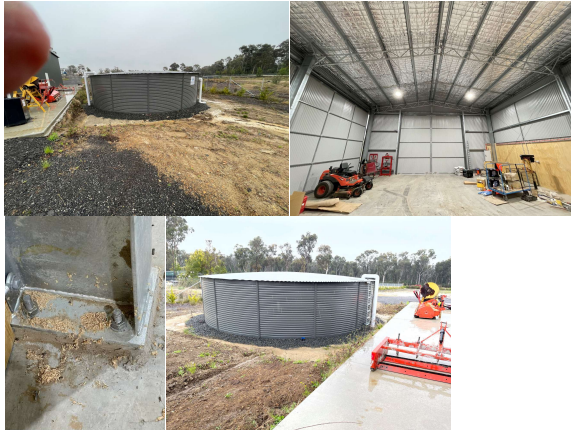
Figure 4 Shed and adjacent rainwater tank structures
