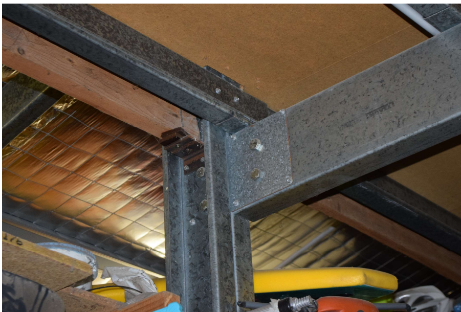
Figure 6 Packing between timber beams and angle seat brackets.
