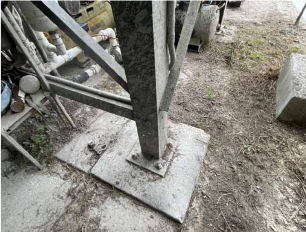
Fig. 3.6 Silo hopper tower bolted connections for baseplates of tower legs
