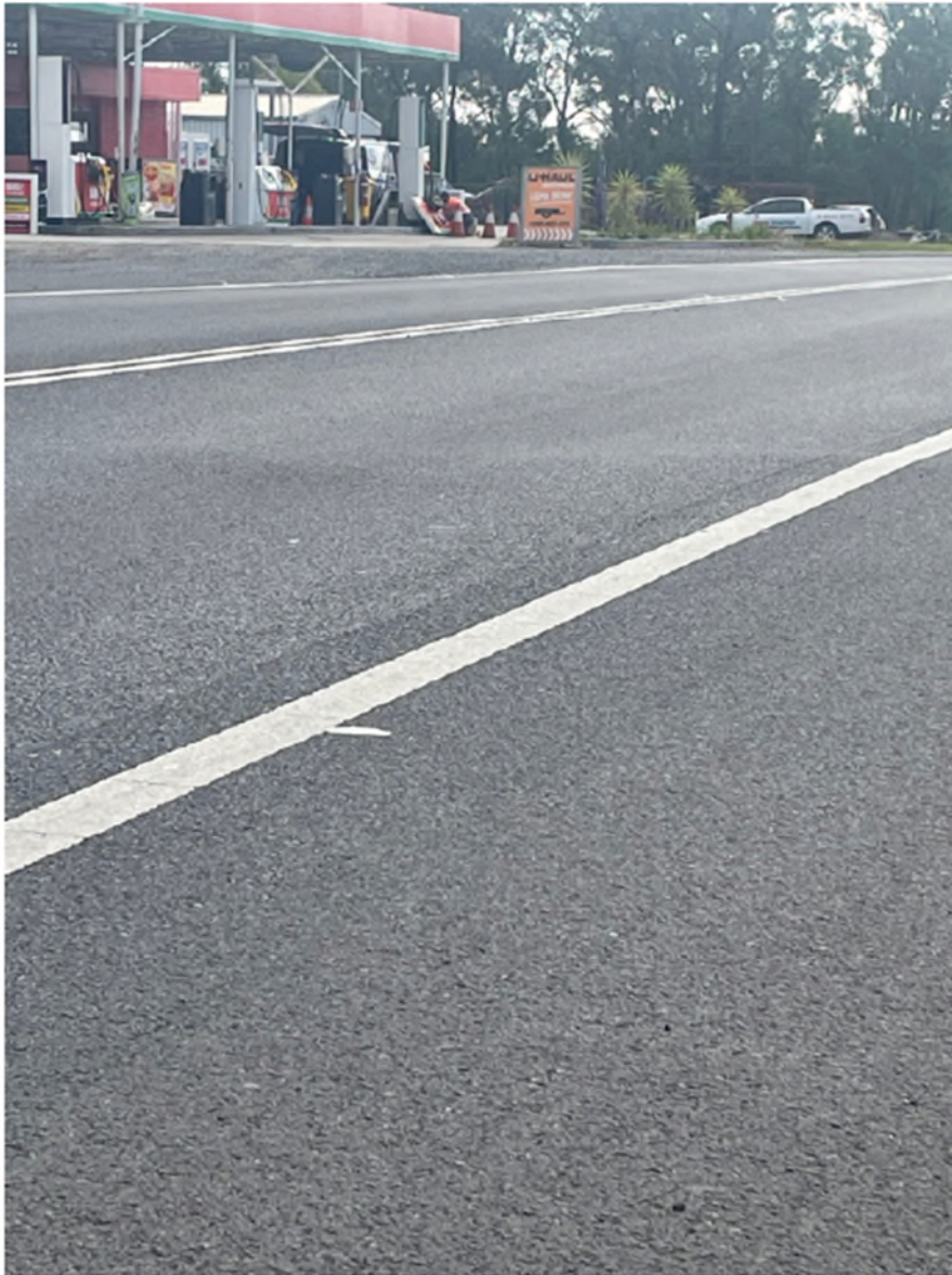
Figure 3-19 Small bump observed in southbound lane of Remembrance Drive near Peg R46 on 31 May 2023 (Source: MSEC1368 Report 19a, Appendix A)
