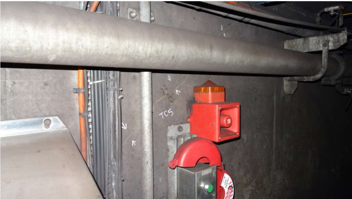
Plate 4.5 Crack C5 (David Talbert, 6 June 2023).
