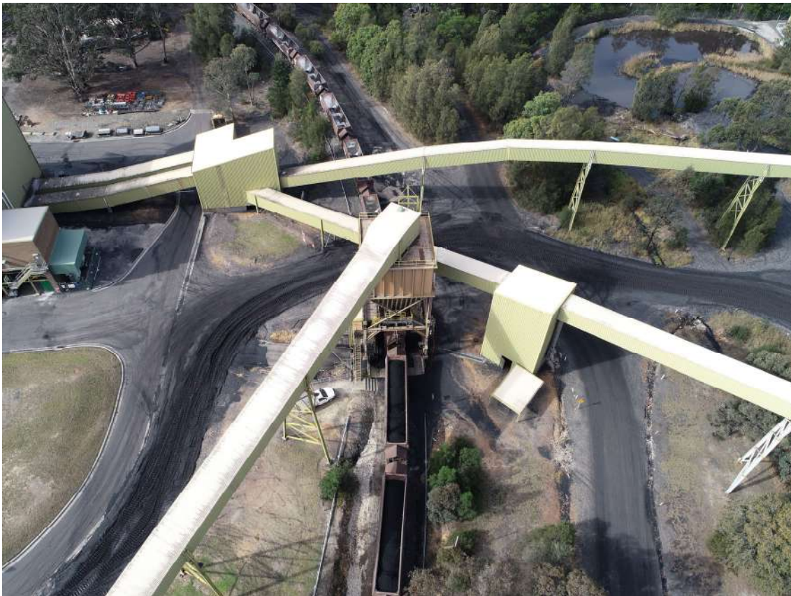
Fig. 6.14 Conveyors 4S and 4C over Rail Loop and Rail Loader Bin
