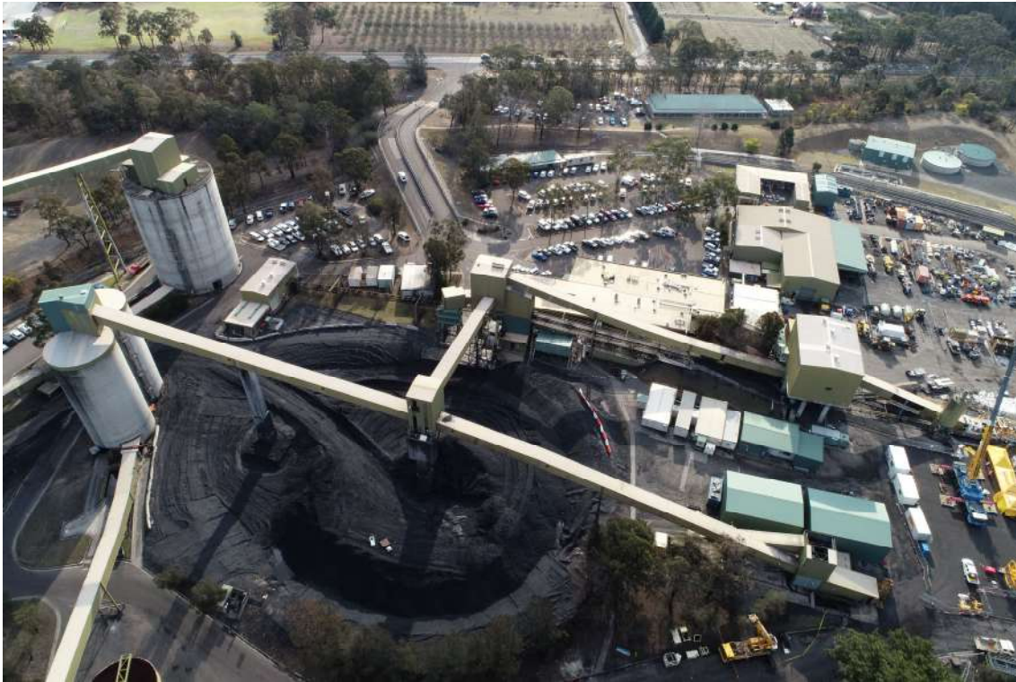
Fig. 9.7 Aerial photograph showing Bins, Raw Stockpile, Drift Portal and Winder
