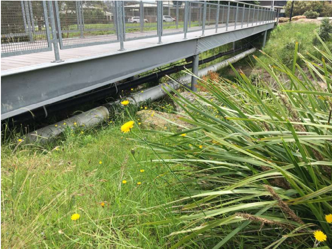
Fig. 7.10 Wollondilly Anglican College – Footbridge
