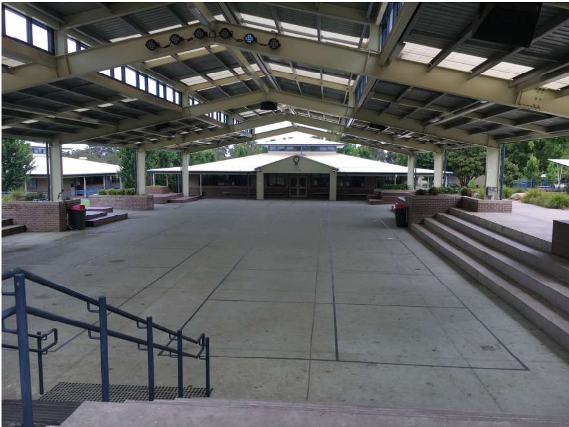
Fig. 7.9 Wollondilly Anglican College – Shoulder to Shoulder Shelter
