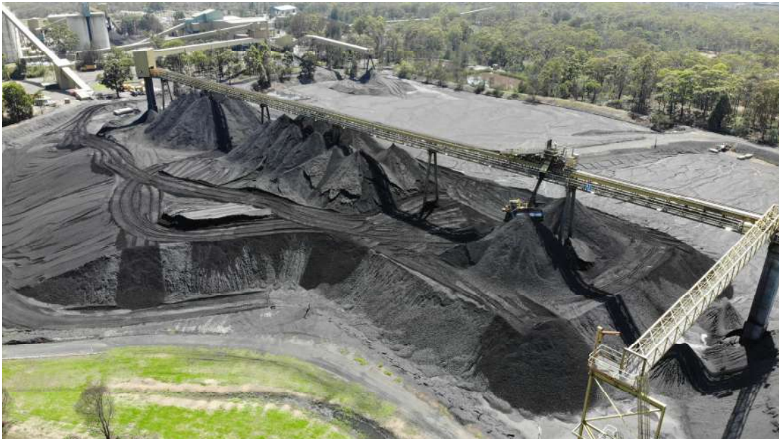
Fig. 9.4 Aerial view of Stockpile area and Overhead Conveyor 5C
