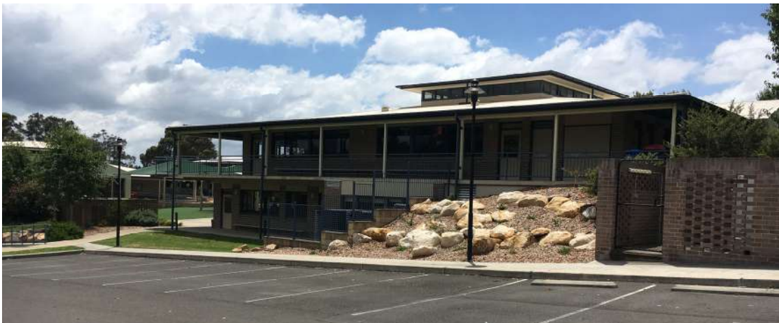
Fig. 7.4 Wollondilly Anglican College – Elizabeth Cottage (two-storey)
