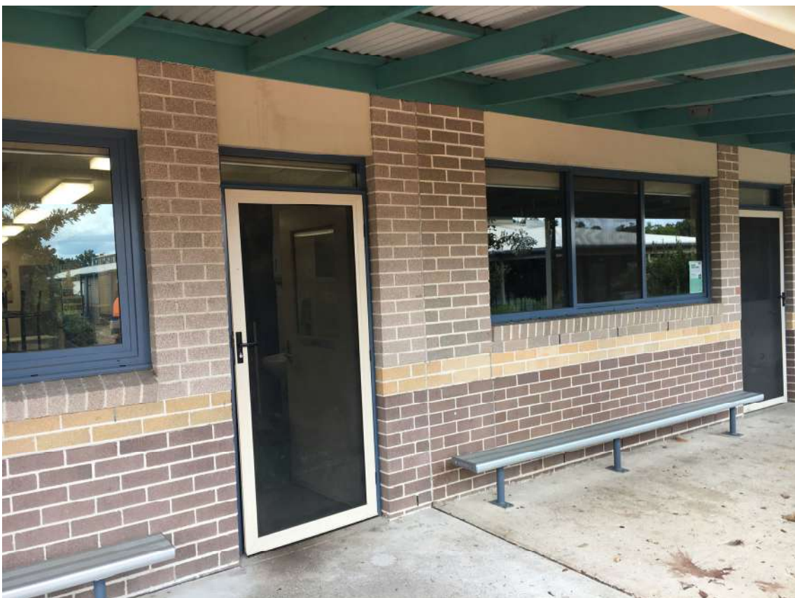
Fig. 7.5 Wollondilly Anglican College – Example of brickwork details
