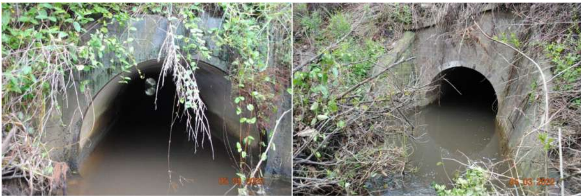
Fig. 6.19 RCP culvert beneath Remembrance Drive and brick arch culvert beneath Main Southern Railway at 100.425 km with private land in between them
