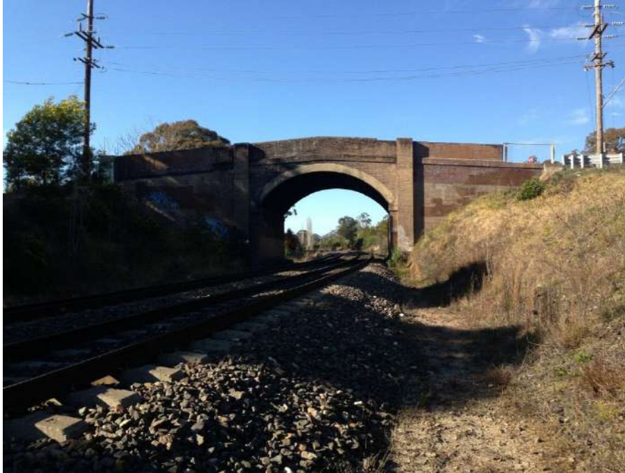
Fig. 6.4 Wellers Road Overbridge at 101.162 km
