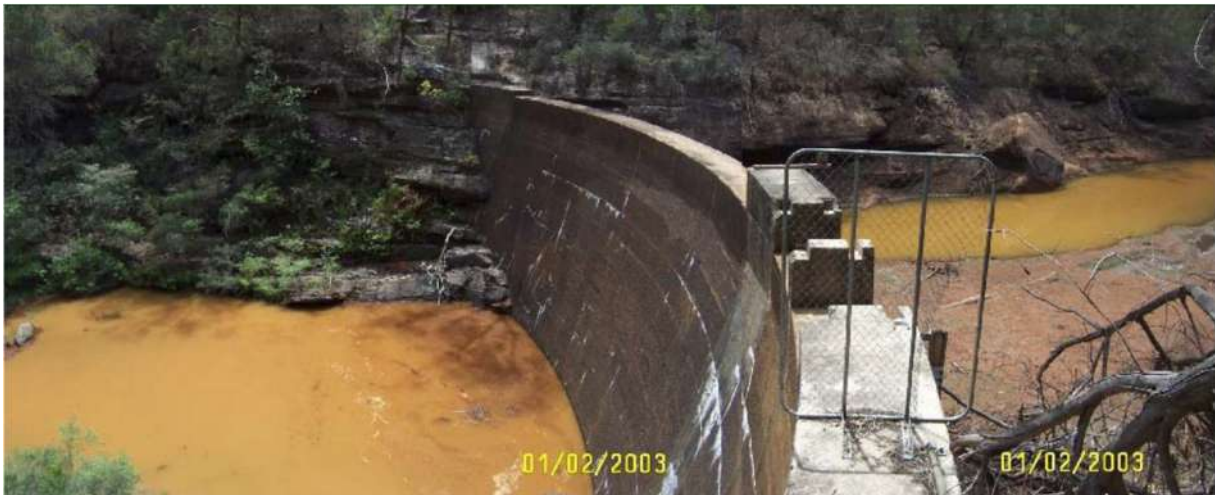
Fig. 5.10 Picton Weir 1 st February 2003
