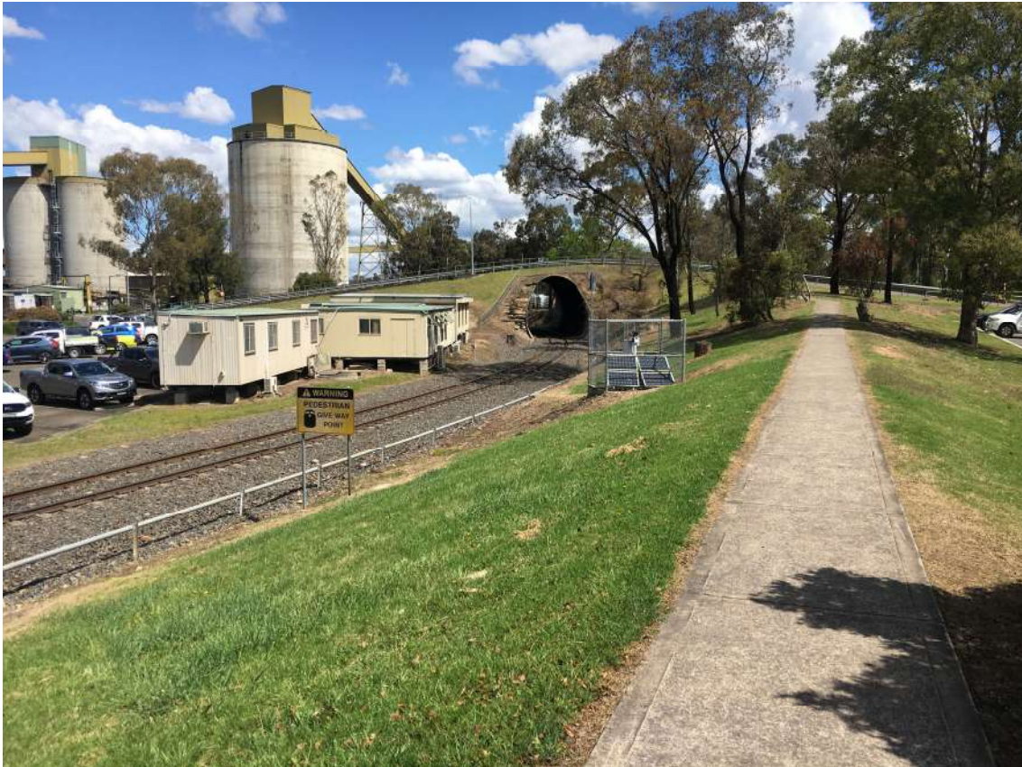
Fig. 6.12 Rail Loop under road bridge
