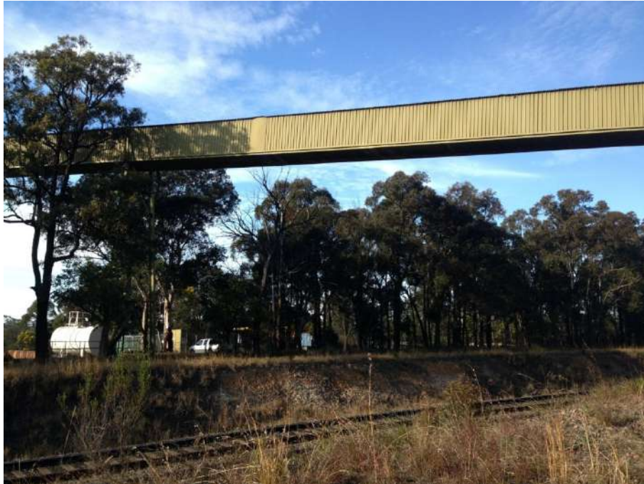
Fig. 6.3 Tahmoor Mine overhead coal conveyor 3R over the Main Southern Railway near 98.160 km
