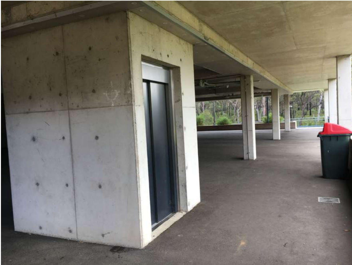
Fig. 7.8 Wollondilly Anglican College – Lift in Cuthbert Cottage
