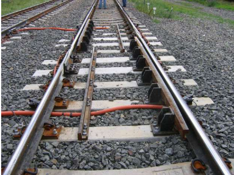
Fig. 6.2 Rail expansion switch
