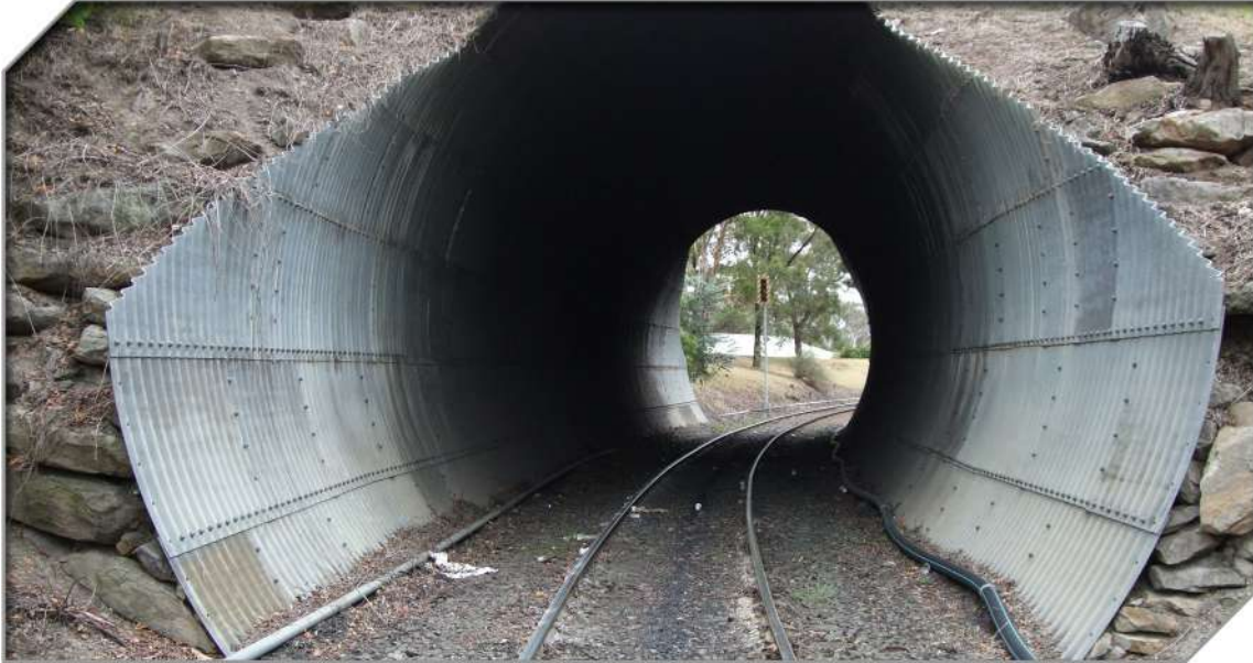
Photograph courtesy JMA Solutions
