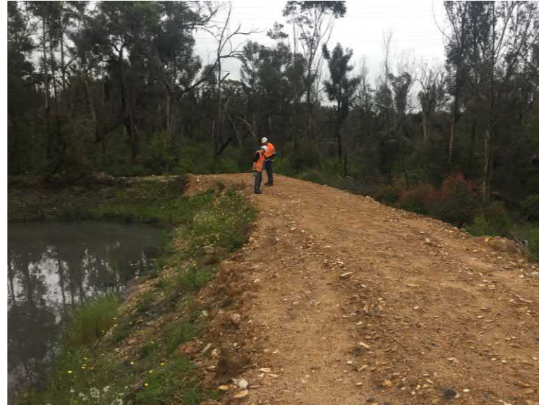
S9 East Bank Looking North
