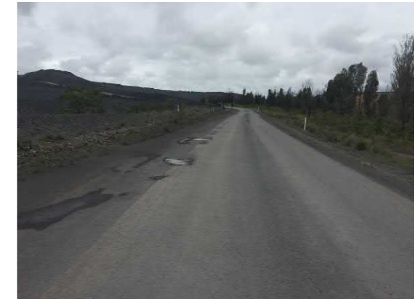
S7 Western Embankment Crest
