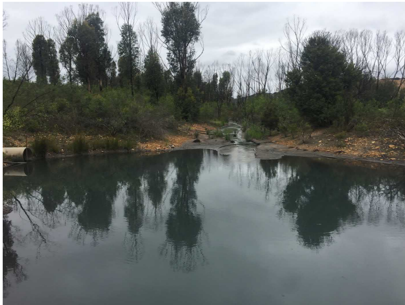
S7b Looking South at channel inlet from S7
