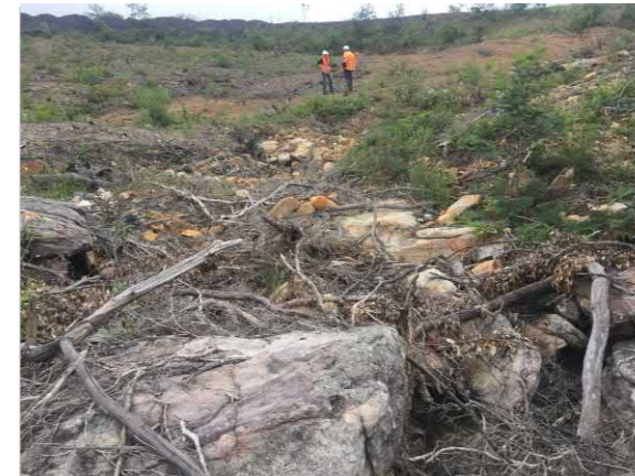
Remnant Gully downstream of S7a Western Embankment
