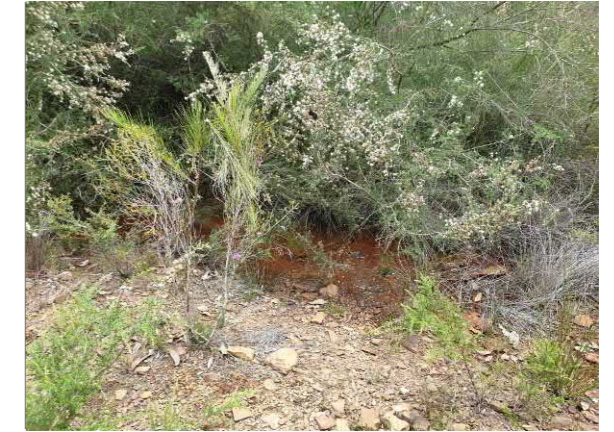
M6 Downstream Seepage
