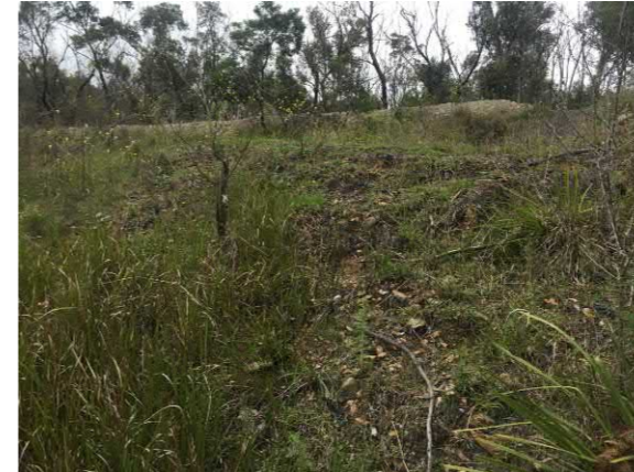
S10 Eastern Road Embankment
