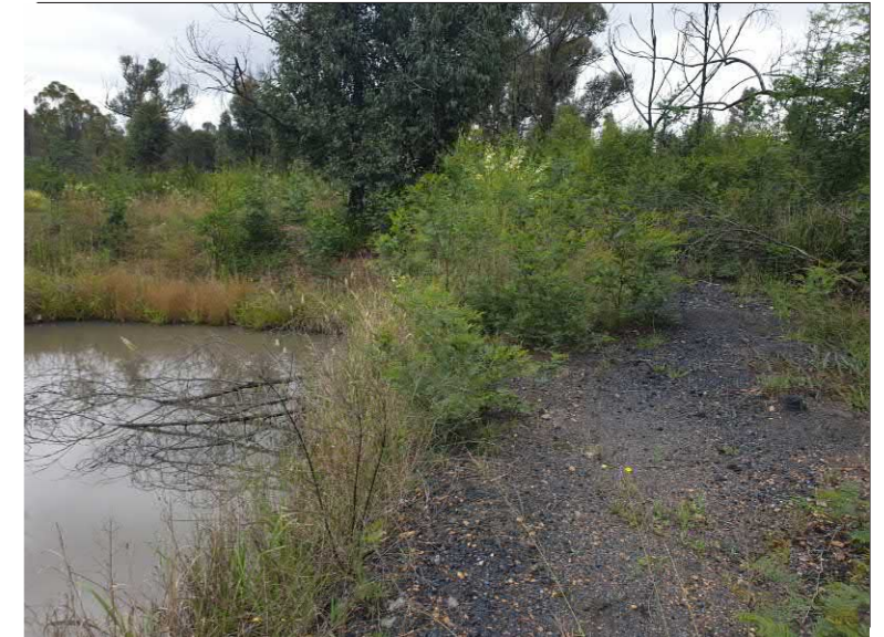
S5 Eastern Embankment Looking North
