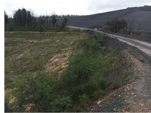
S7a Western Embankment Downstream
