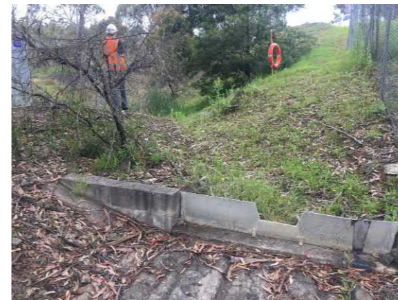
S9 Spillway NW Corner
