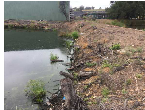
Embankment Between STP1 and SPT2
