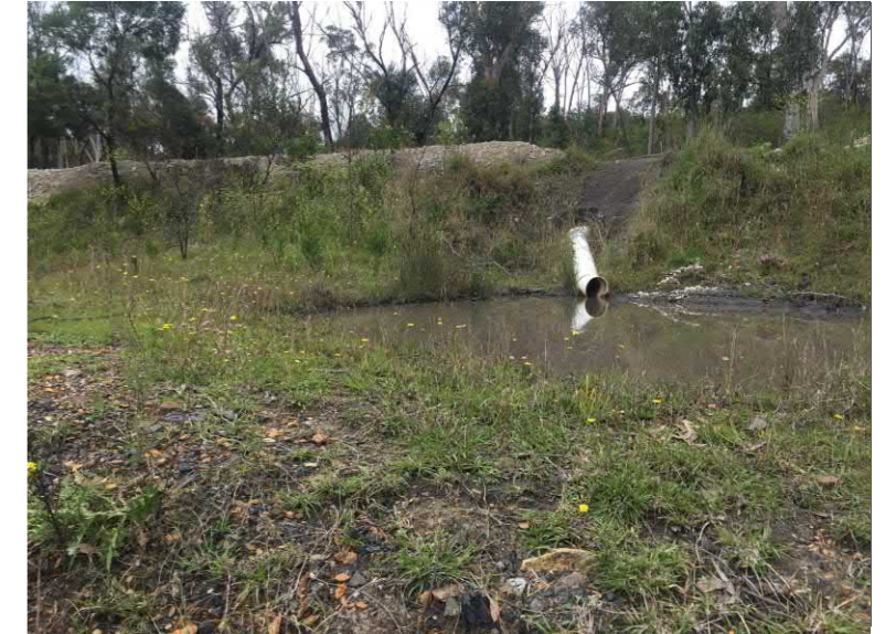
S10 Looking North East
