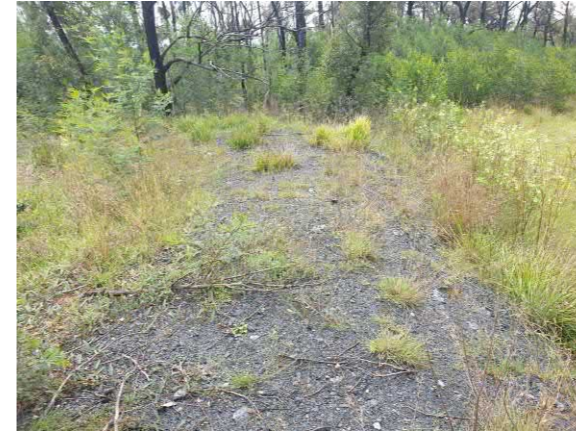
S5 Northern Embankment Crest
