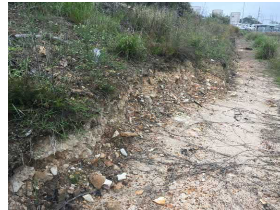
M4 Embankment Conditions
