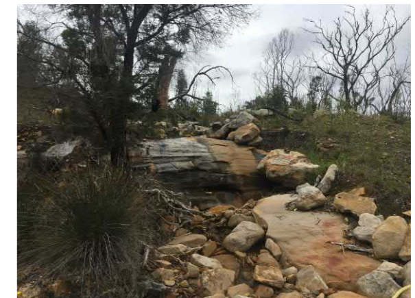
S8 Channel Inlet
