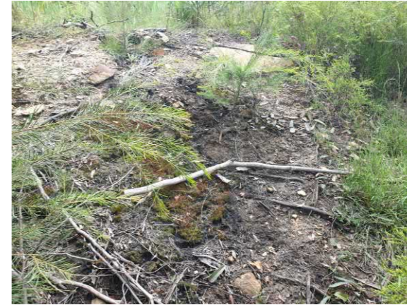
S6a Northern Embankment Downstream
