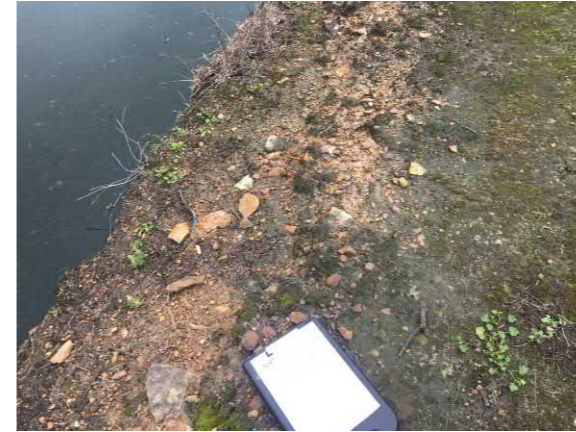
STP Foundation Conditions
