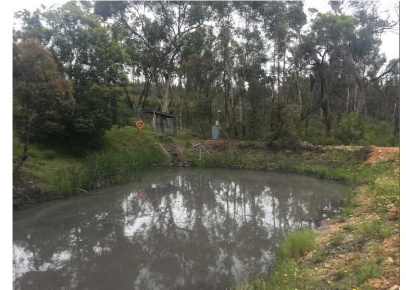
S9 East Embankment Looking West
