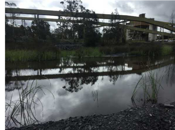
S2 & S3 Embankment + Foundation Conditions
