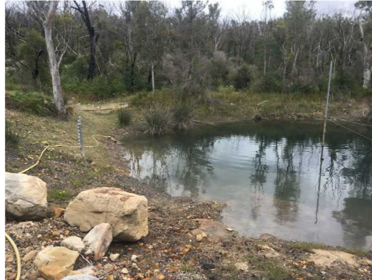
S8 East Bank Looking West at Spillway
