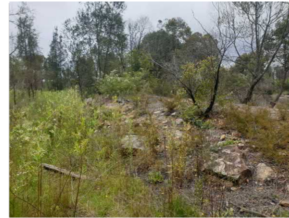
S6 Looking North East, Downstream Western Embankment
