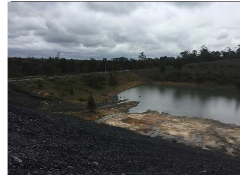
S7 Southern Embankment Looking North West
