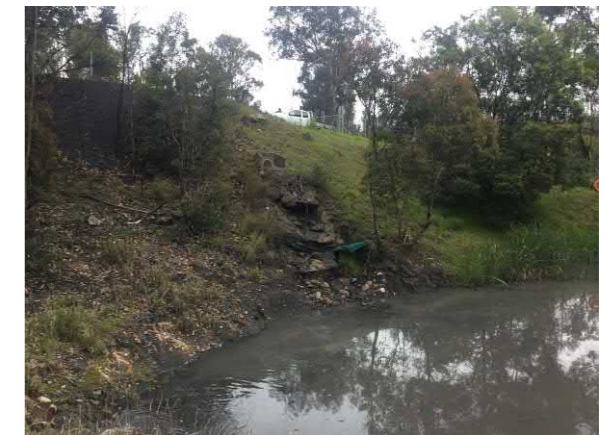
S9 Southern Embankment
