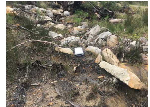
S8 Downstream of Spillway
