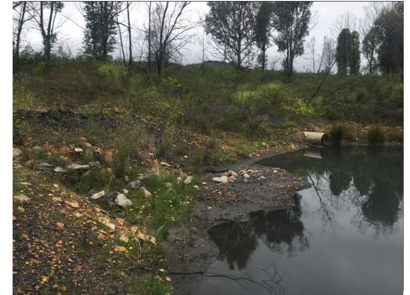
S7b Northern Embankment Looking South East
