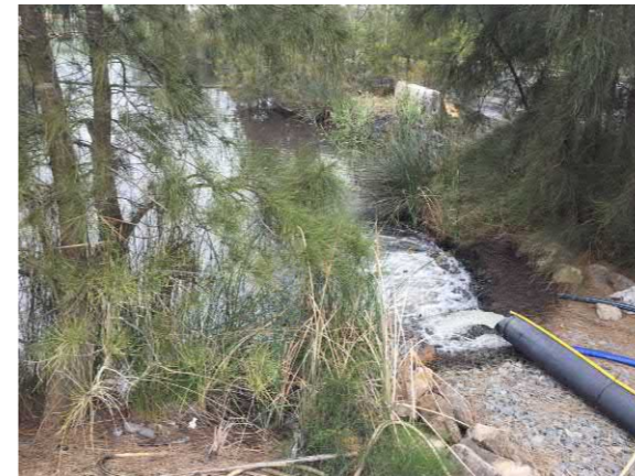
M3 Foundation Conditions
