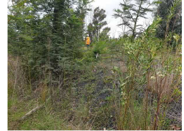
S5 Downstream NE Embankment
