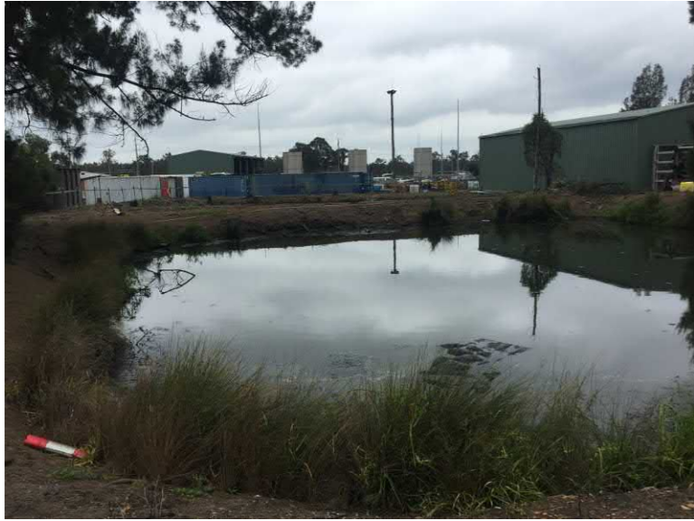
STP1 Looking North
