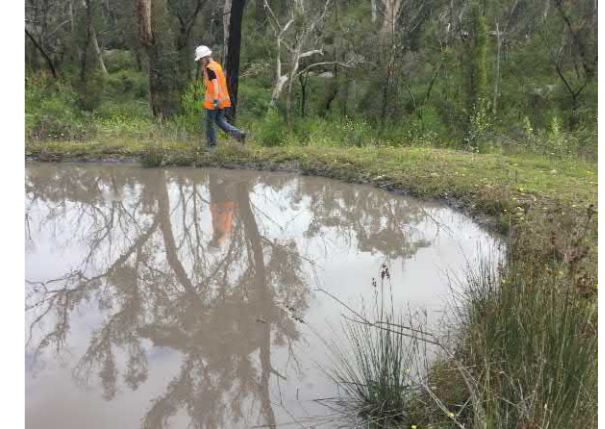
S10 Western Embankment
