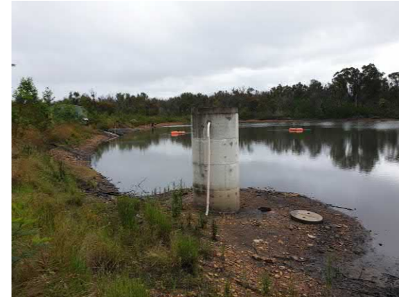
S4 Embankment + Foundation Conditions
