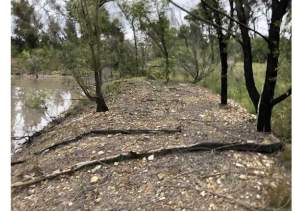
S6 Western Embankment Looking South West
