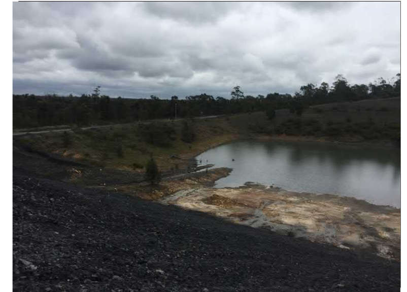
S7a Southern Embankment Looking North West
