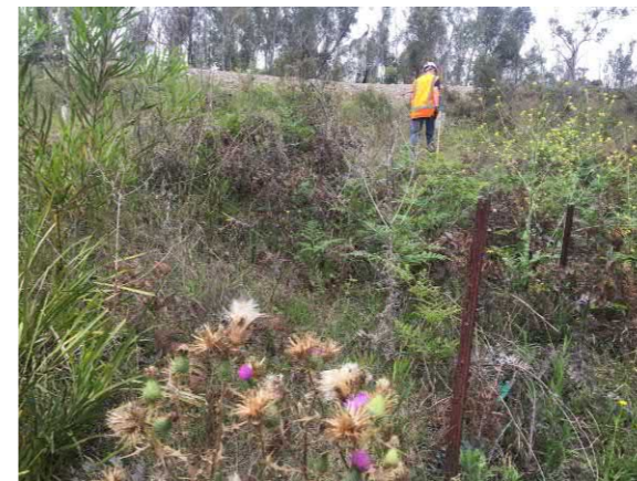
S10 Downstream Embankment
