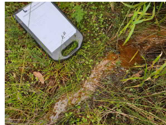
S4 Downstream Seepage
