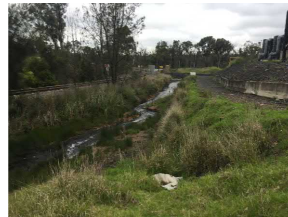
M4 Downstream Spillway Runoff
