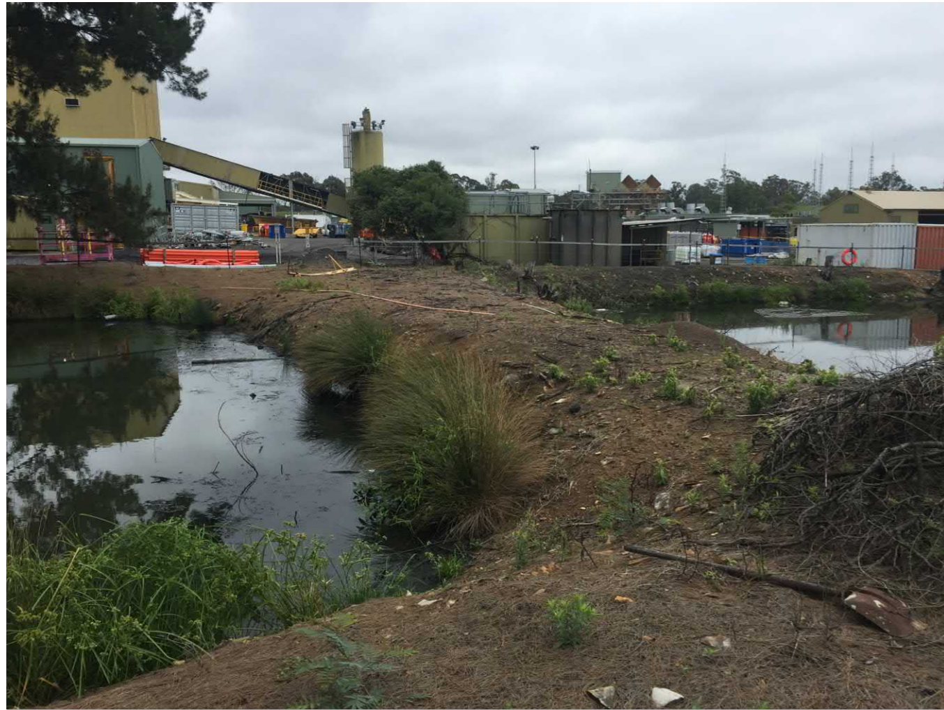
STP1 & STP2 Looking West
