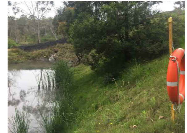
S9 Southern Embankment Looking East
