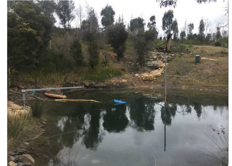
S8 Northern Embankment Looking South
