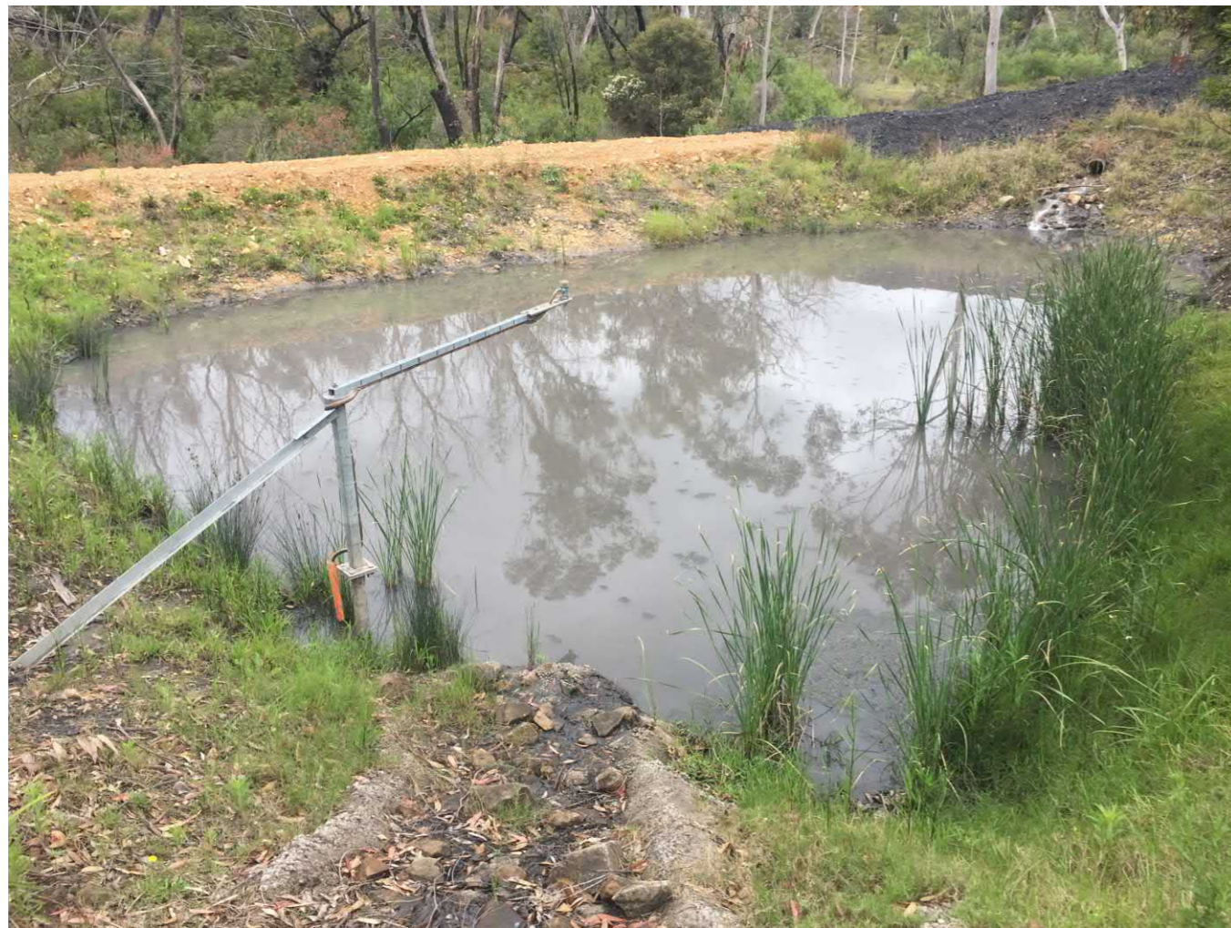
S9 Looking East
