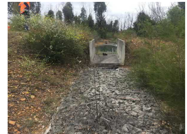
S7b Spillway outlet
