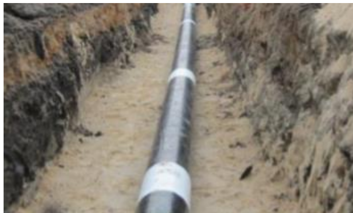
Figure 6 – Pipe exposed or ‘uncoupled’ to eliminate potential ground strain
