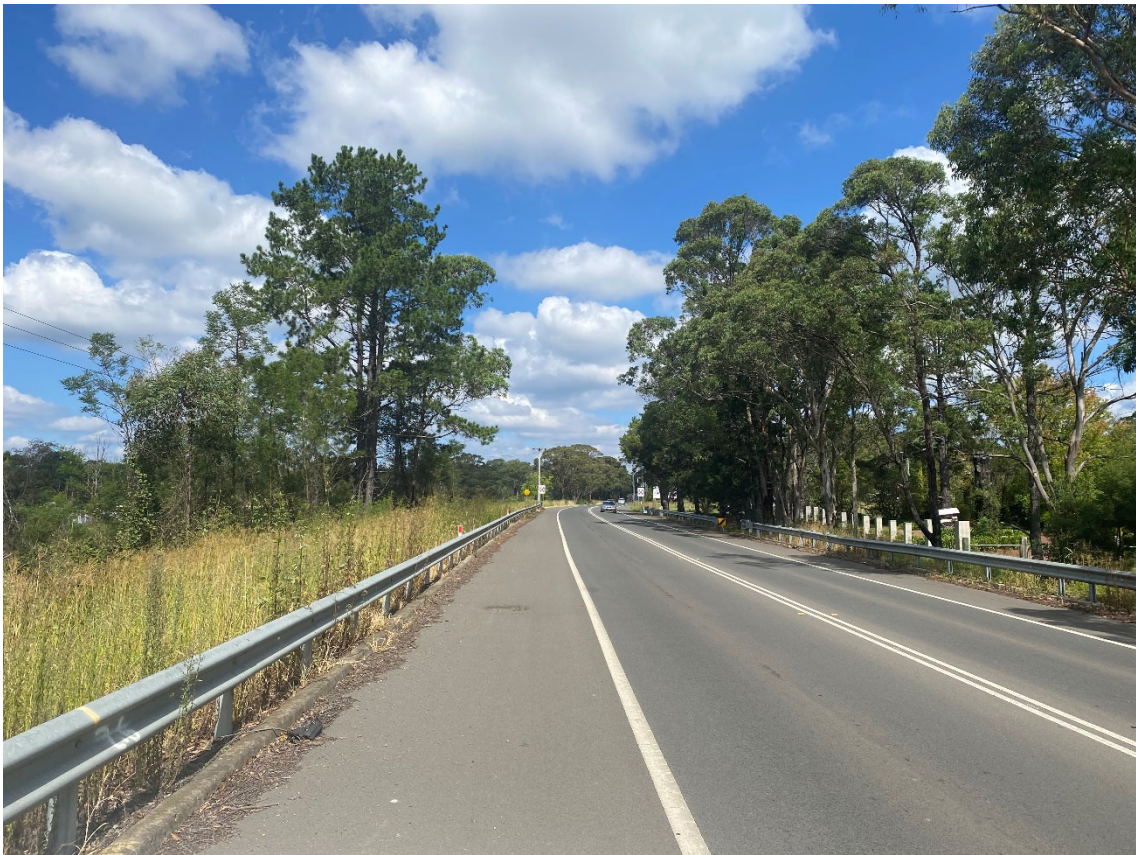
Fig. 3.20 Remembrance Drive embankment south of Yarran Road on southbound side
