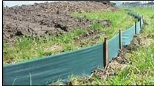
Figure 20 – Typical Sediment Control Fence
