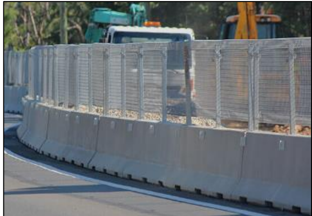
Figure 7 - Barrier with gawk screen high hoarding
