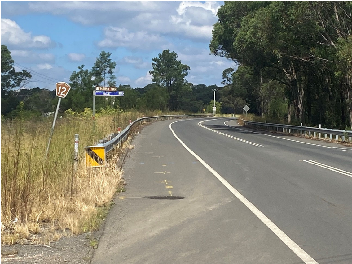
Fig. 3.19 Remembrance Drive embankment south of Yarran Road on southbound side
