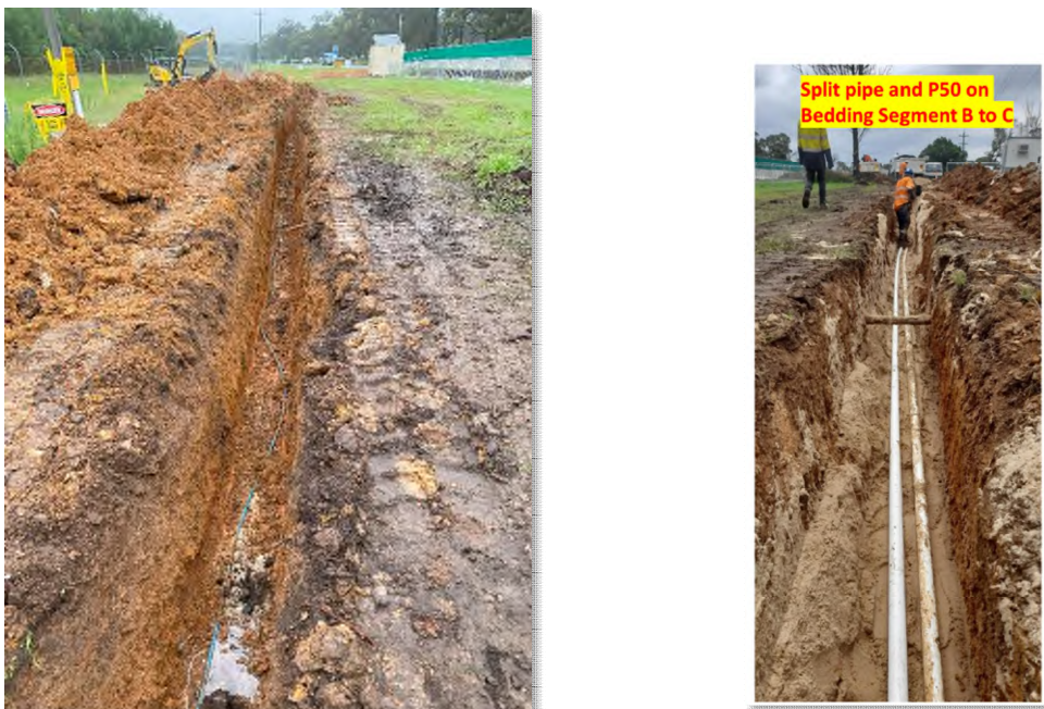
Figure 9 Excavation and protection of optic fibre cable along Remembrance Drive (Jan 2024)
