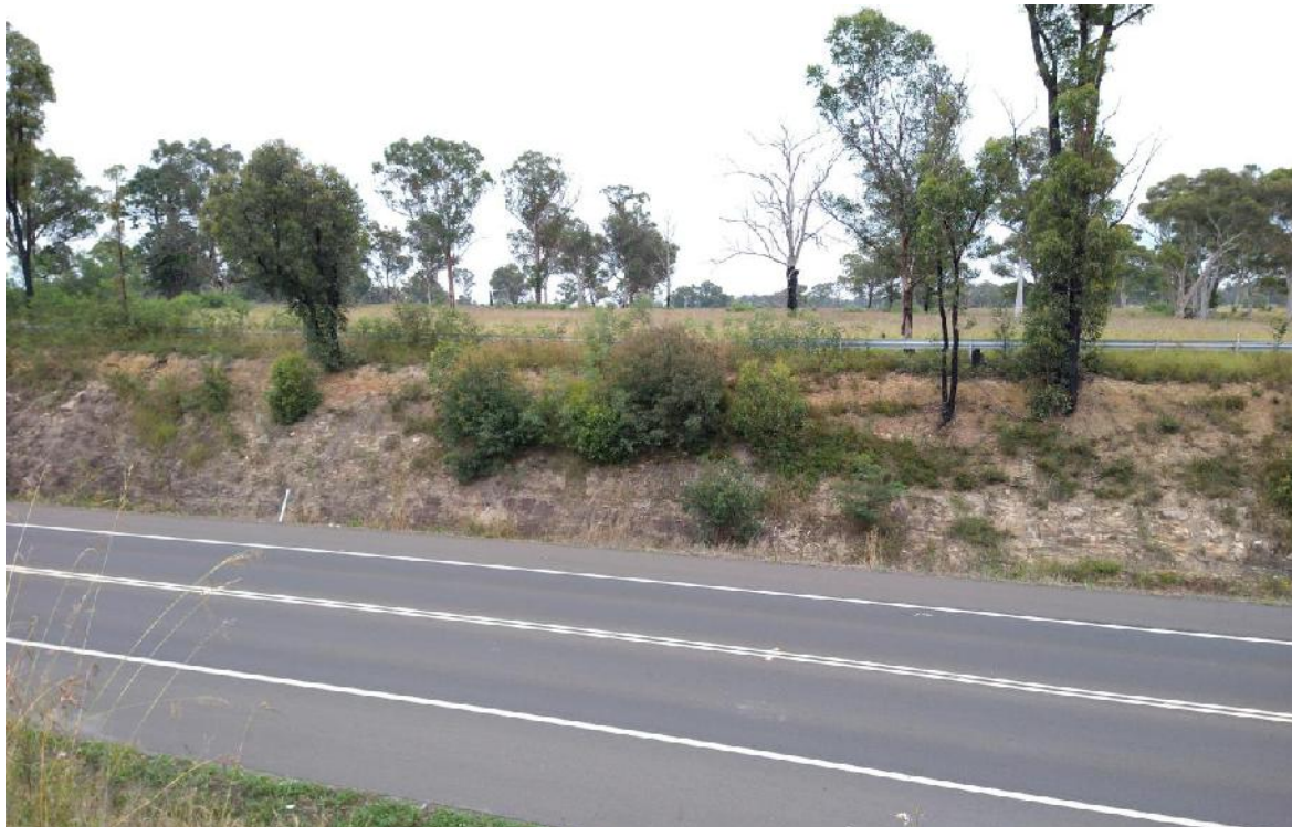
Photo 13: View looking southwest towards the road cutting adjacent to No. 3140 Remembrance Drive. Note: the soil and weathered rock in the upper cut and medium to thickly bedded rock in the middle and lower.
