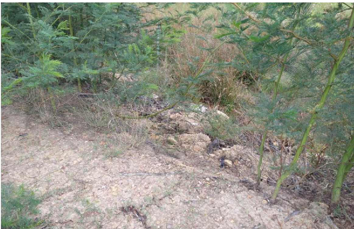
Photo 40: View looking at erosion in the downstream embankment face of FD31. Note: the saplings growing in the downstream face.
