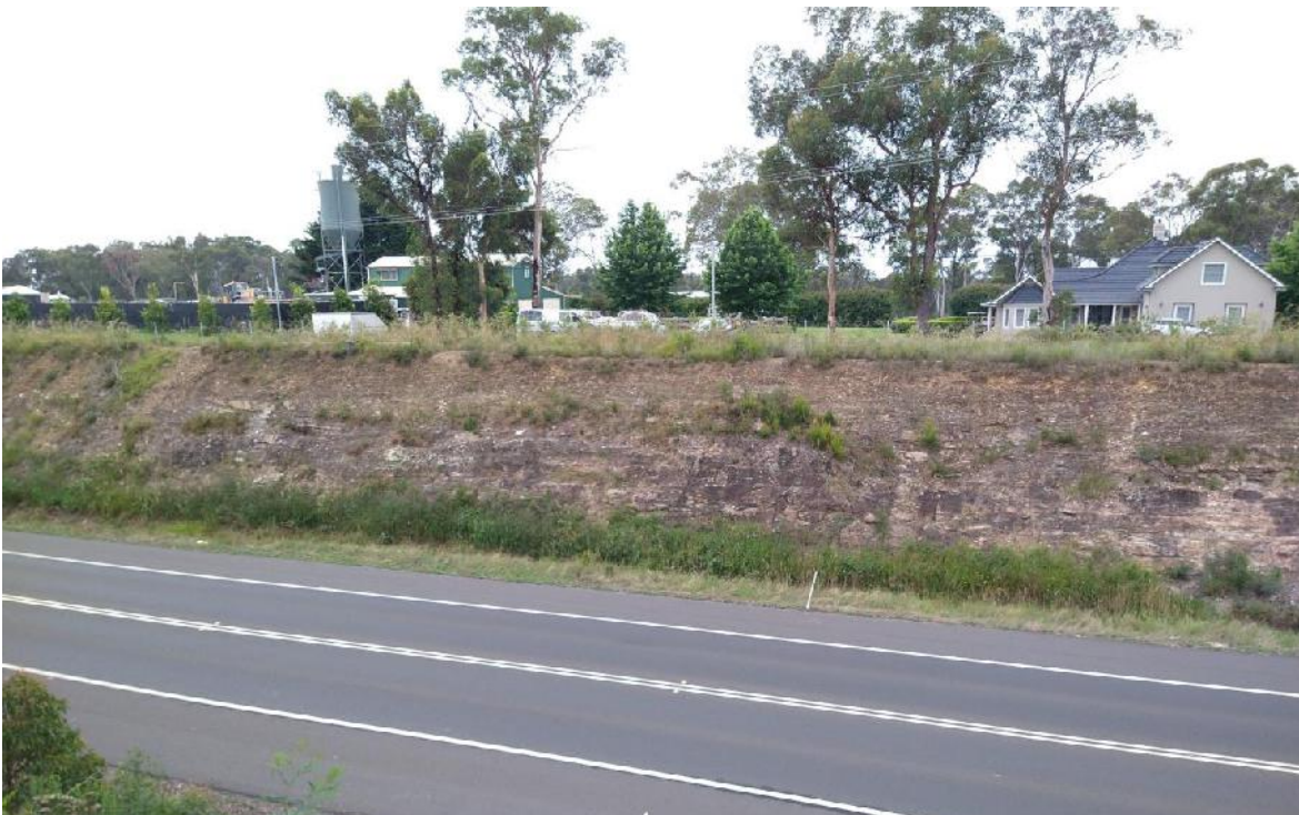
Photo 15: View looking east towards the cutting adjacent to No. 3165 Remembrance Drive. Note: the weathered rock in the upper cut and medium to thickly bedded rock in the middle and lower cut.
