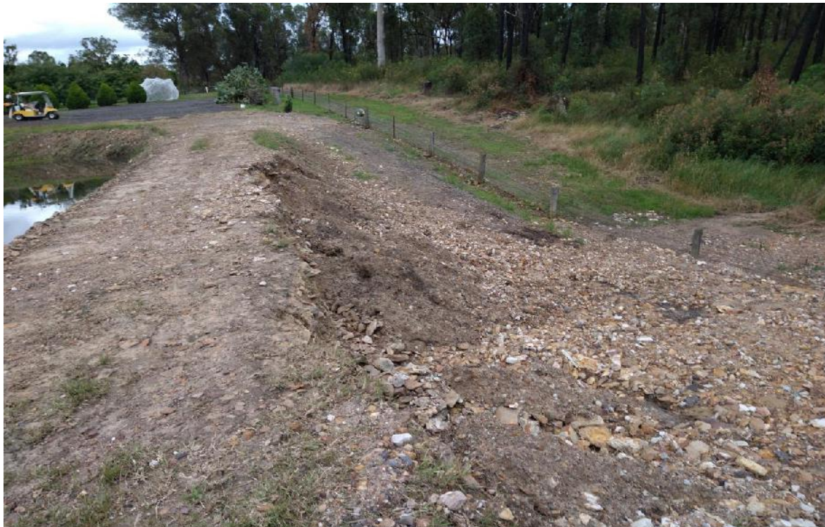
Photo 25: View looking west along the crest of the farm dam at 4 Olive Lane (ie outside SA). Note: the erosion and scour following overtopping during a heavy rainfall event in early April 2022.
