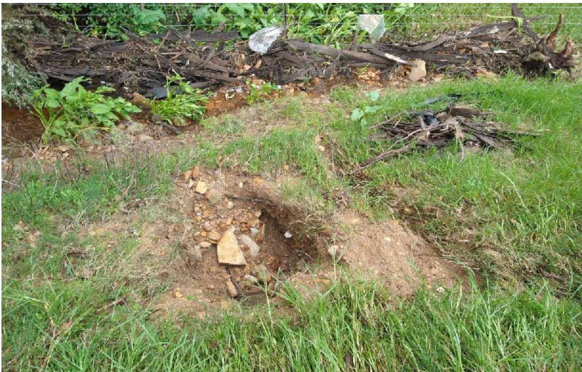
Photo 38: View looking at erosion and scour in the downstream face of FD27. Note the spillway channel at the toe of the embankment in the upper photo.
