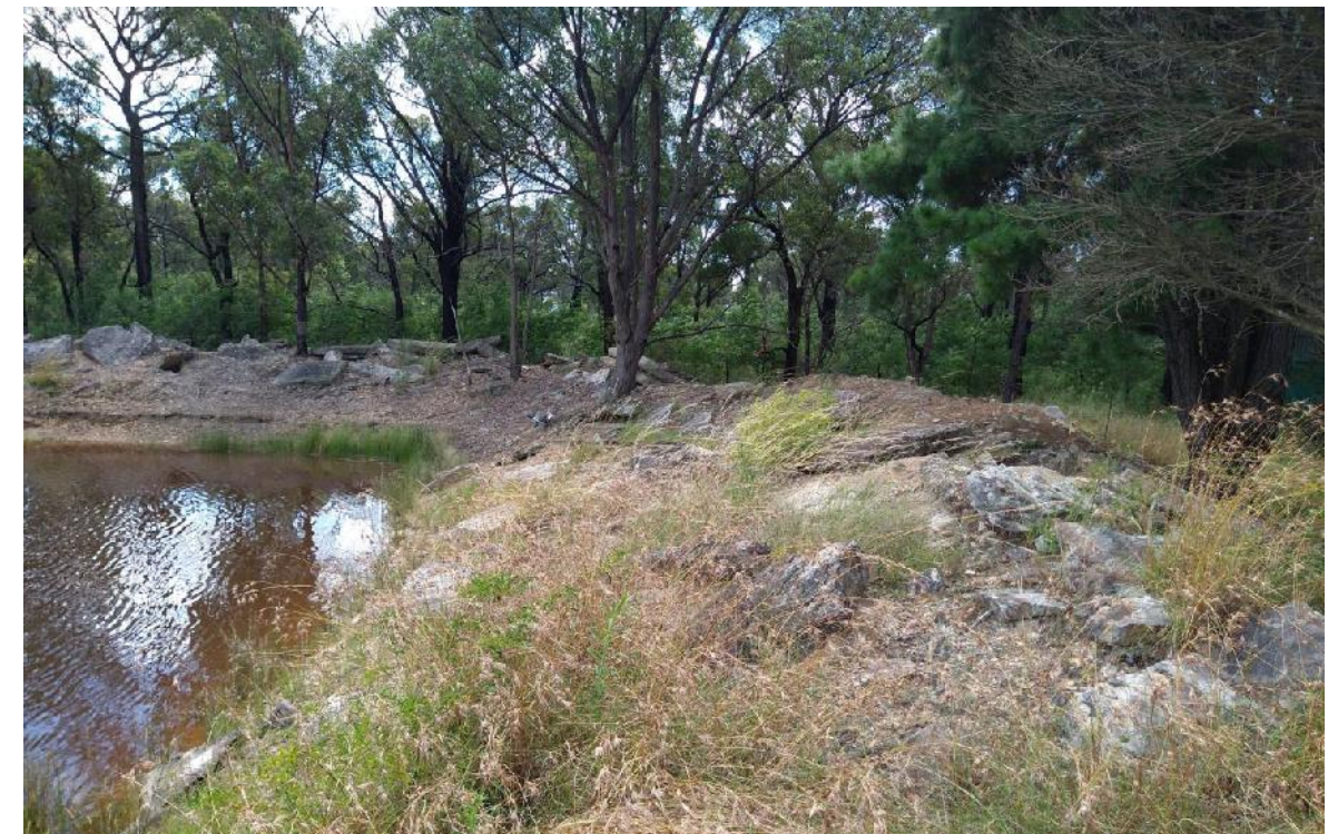
Photo 32: View looking north along the crest and upstream embankment face for FD8. Note: the large sandstone boulders placed over the crest.
