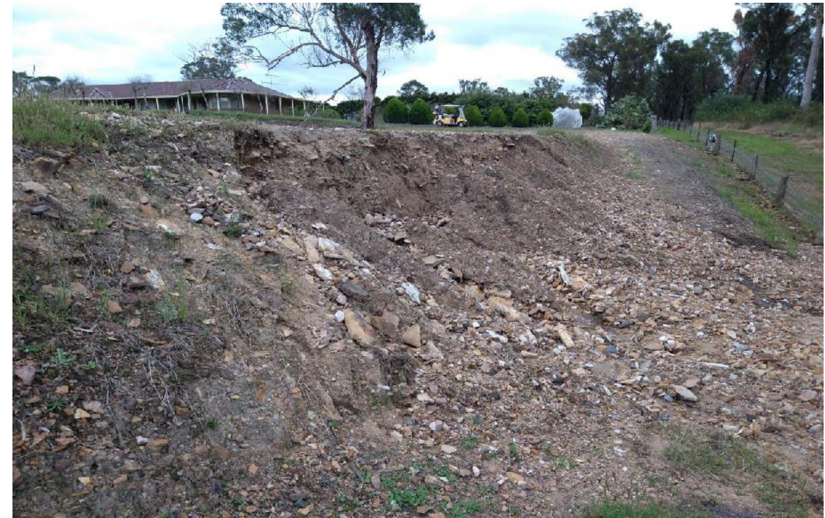
Photo 26: View looking west along the downstream toe of the farm dam at 4 Olive Lane (outside the SA). Note: the erosion and scour following overtopping during a heavy rainfall event in early April 2022.
