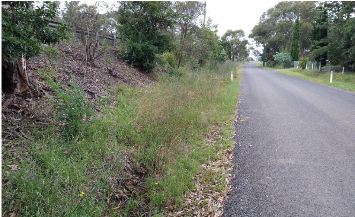
Photo 11: View looking south along the upstream face of RE4 opposite No. 3100 Remembrance Drive. Note: the drain cut into the toe of the embankment.
