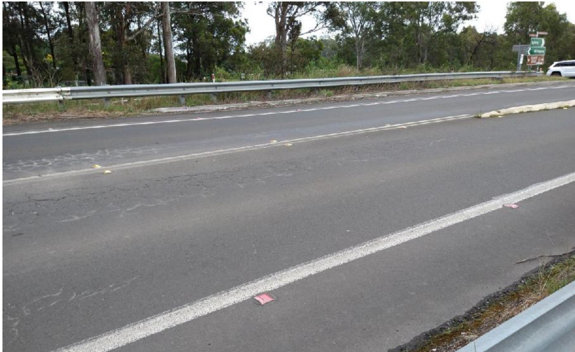
Photo 3: View looking north west at rutting and crocodile cracking in the Remembrance Drive wearing course to the south of the intersection with Wellers Road (RE1).
