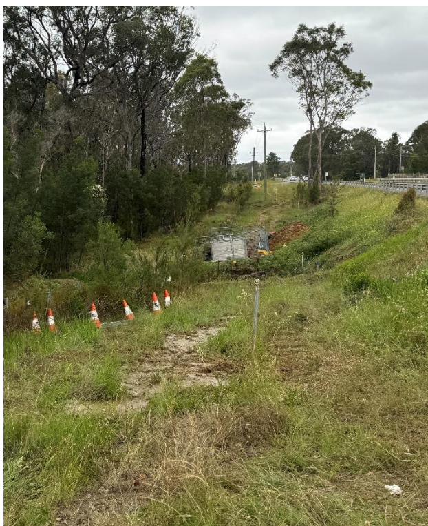
Figure 2 View of Creek 2 excavation site to install joints
