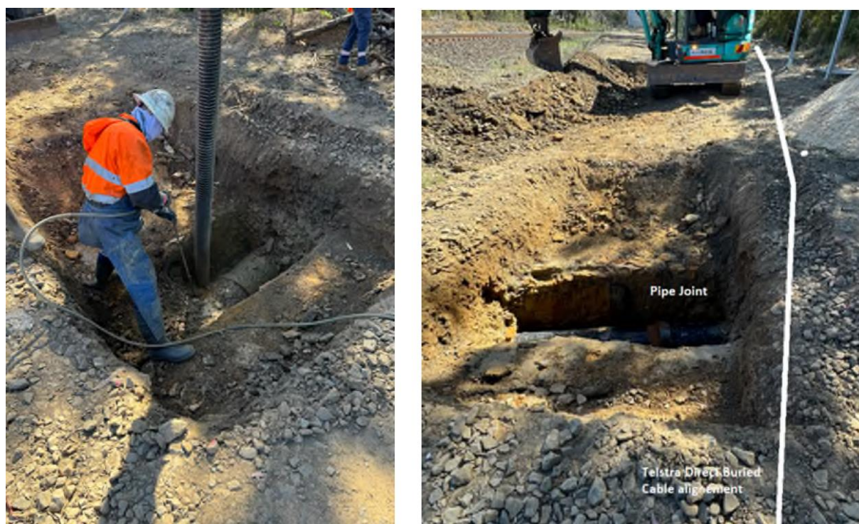
Figure 7 Exposed CICL water main on eastern side of Railway crossing (Down side)
