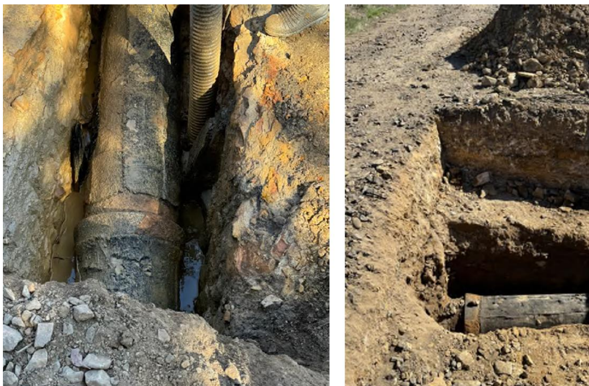
Figure 6 Exposed CICL water main on western side of Railway crossing (Up side)
