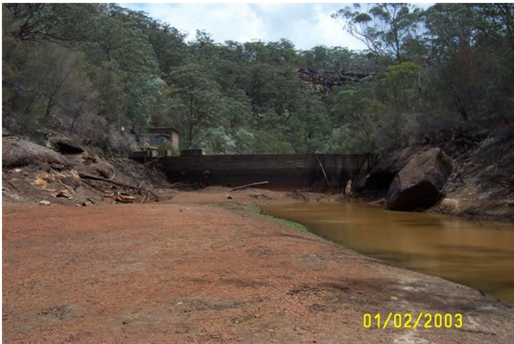
Fig. 1.6 Silt levels behind Picton Weir in February 2003
