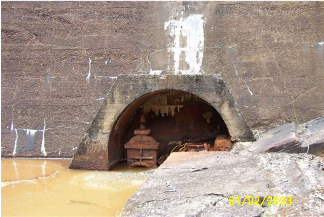
Fig. 1.5 Seized open valve and outlet pipe at base of Weir
