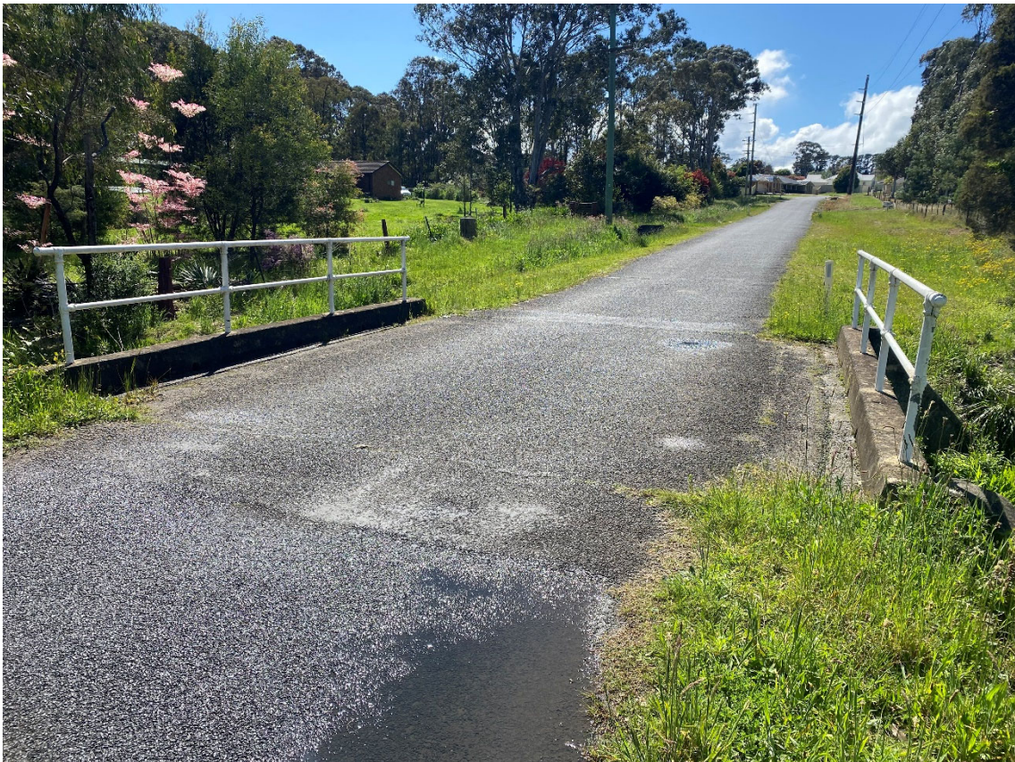
Fig. 3.61 Kader Street Bridge over Hornes Creek from western approach road
