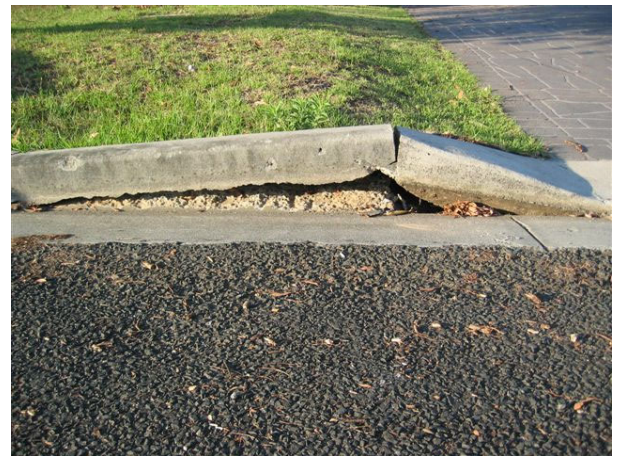
Fig. 3.24 Impacts on local roads above Tahmoor Mine
