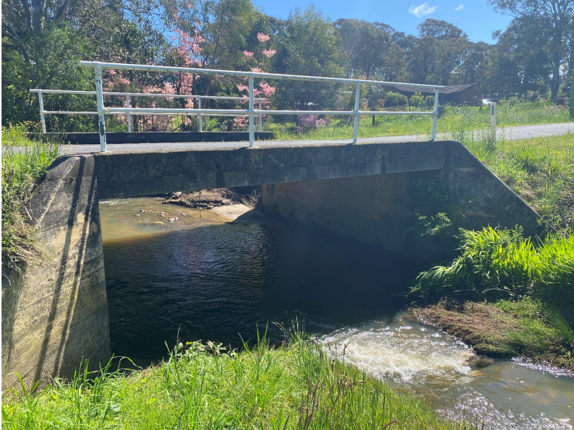
Fig. 3.60 Kader Street Bridge over Hornes Creek from upstream side
