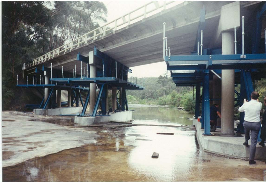
Fig. 3.46 Jacking frames installed at Rockford Road Bridge over Bargo River
