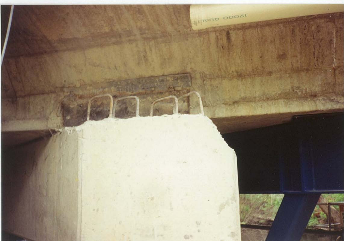
Fig. 3.45 Headstock bents / upstands removed at Rockford Road Bridge prior to mining of LW12
