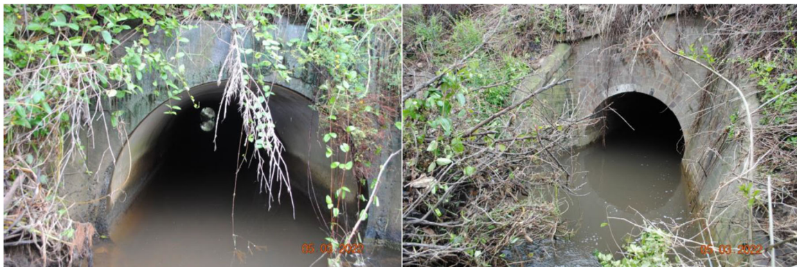
Fig. 3.26 RCP culvert beneath Remembrance Drive and brick arch culvert beneath Main Southern Railway at 100.425 km with private land in between them
