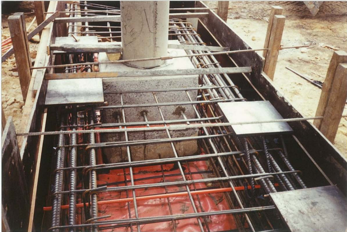
Fig. 3.44 Pad footings tied together at Rockford Road Bridge prior to mining of LW12
