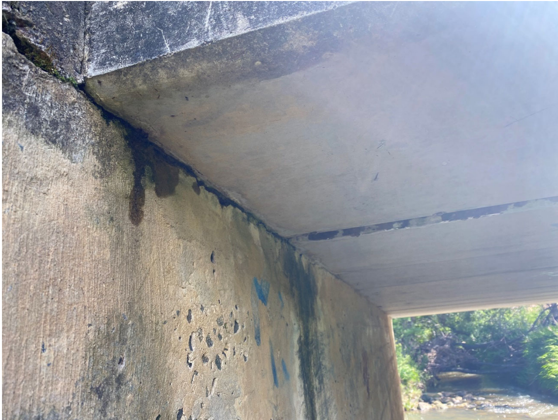
Fig. 3.63 Bridge deck and abutment of Kader Street Bridge over Hornes Creek
