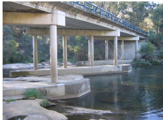
Modified Bridge (post mining in 1994)
