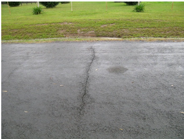
Fig. 3.24 Impacts on local roads above Tahmoor Mine
