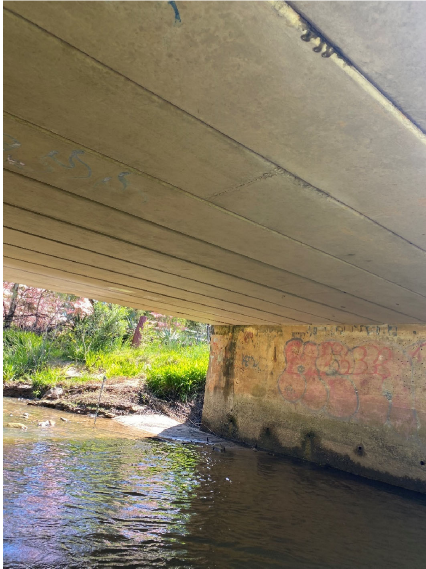
Fig. 3.62 Underside of bridge girders at Kader Street Bridge over Hornes Creek
